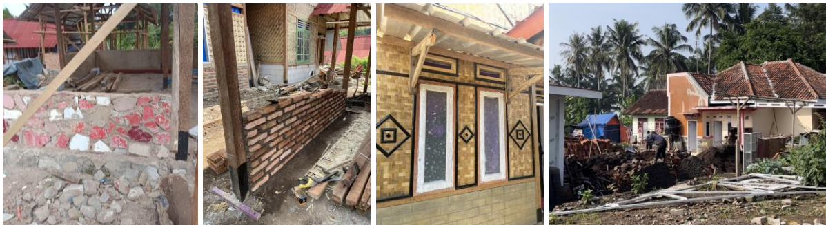
Figure 5 Application of Disaster Waste Material in Recycle House Program and Residents Houses
