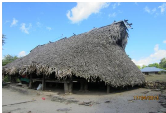
Figure 2 Ammu Hawu traditional house (Suwantara & Rusli, 2013)
