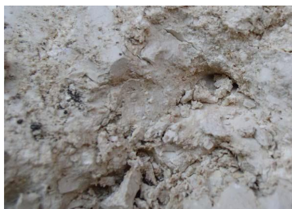
Figure 6 Earth slaked lime with a very firm consistency
