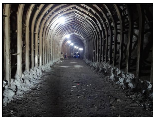
Figure 2 Pandan Duri tunnel constructed in volcanic breccia rock mass
