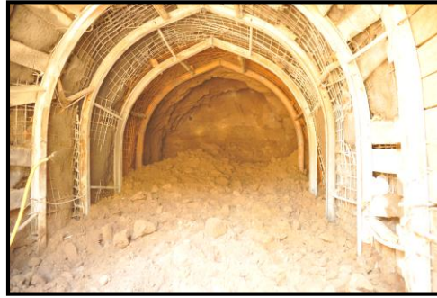
Figure 3 Mila tunnel was excavated into tuff sandstone
