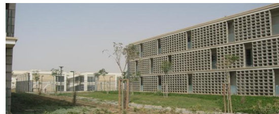
Figure 3 Latticework panels in front of windows
