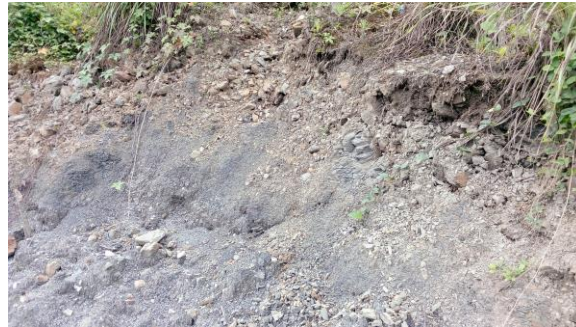
Figure 3 Physical Condition of Weathered Clay Shale in Sentul, West Java
