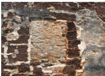
Figure 8 Bricks for stone replacement
