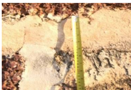
Figure 10 Repointing technique used on St. Paul's Church (50–100mm thick)
