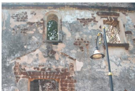
Figure 9 Mortar patching over the laterite wall surface
