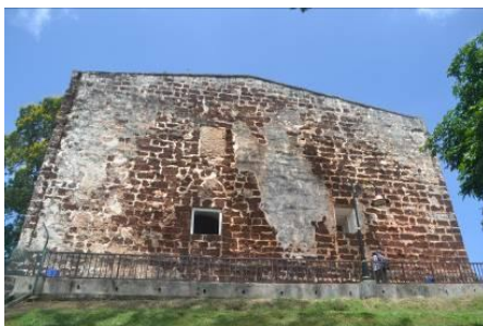
Figure 4 St. Paul's church, Melaka, Malaysia
