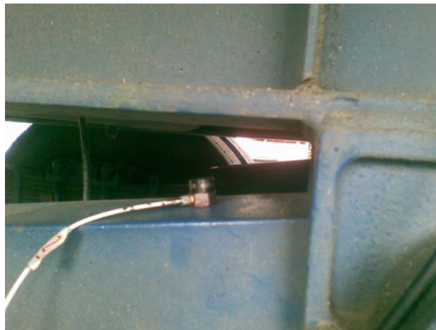
Figure 6 Accelerometer installation on the truck chassis
